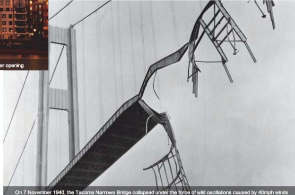
On 7 November 1940, the Tacoma Narrows Bridge collapsed under the force of wild oscillations caused by 40mph winds
